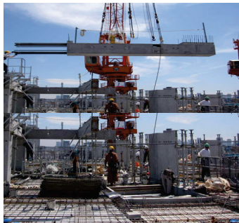
Rapid construction of high-rise building with precast technology
